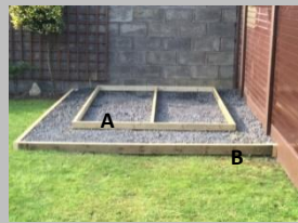
Fig. 1 We supply Sub frame (A) Pressure treated frame is used to contain hardcore but is not supplied by us (B)
