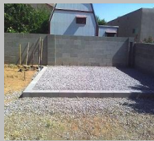
Fig. 2 Hardcore retained by block
